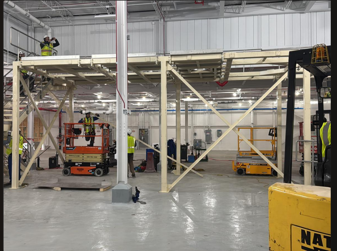
MULTI-LEVEL STEEL STRUCTURES
